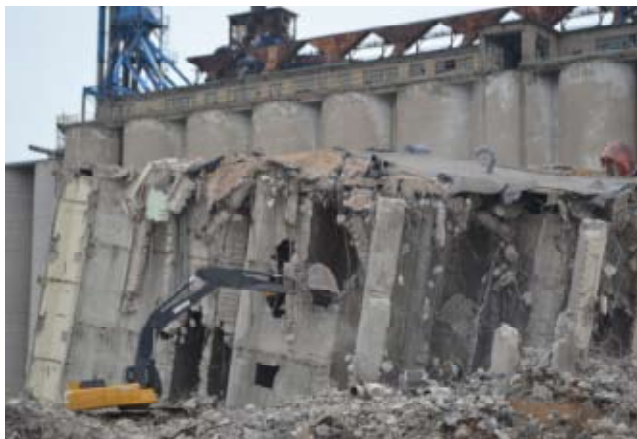
Machinery gnaws away every day on the pile.
