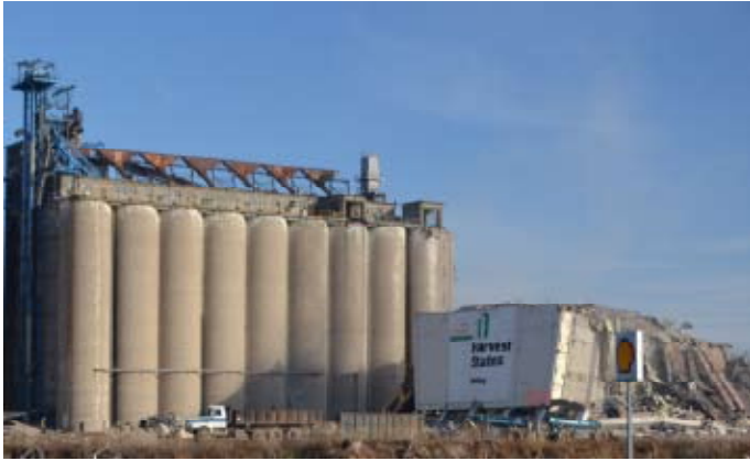
Down for the count, ready for the clean-up
