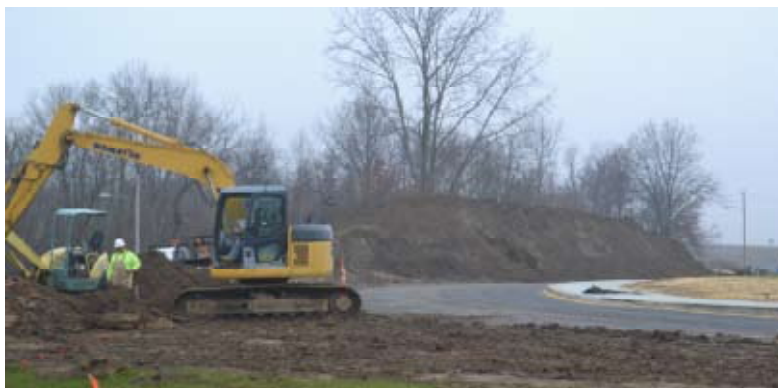
Work continues at Fabens Park improvements.
